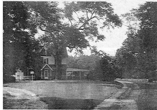
Home of Thornton Phoebus
